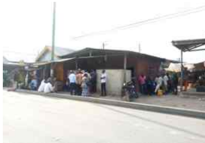
Figure 4: Public toilet at the project site
